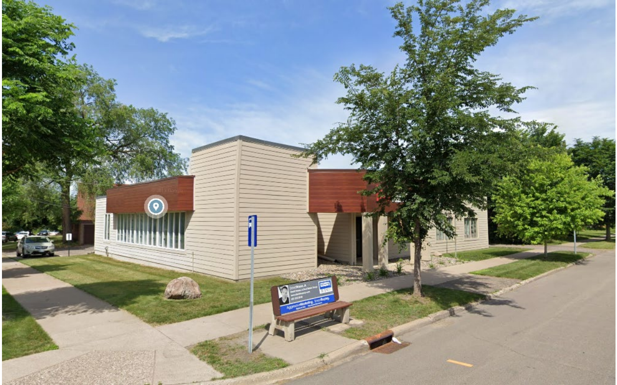
Existing building looking northwest at the corner of Saint Paul Avenue and Saunders Avenue
