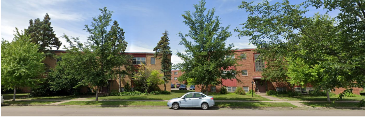
Surrounding multi-unit buildings to the north and west
