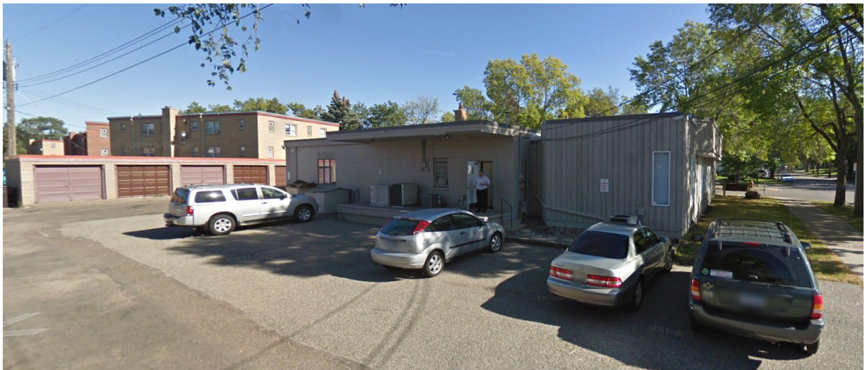
Existing building looking east from the rear alley
